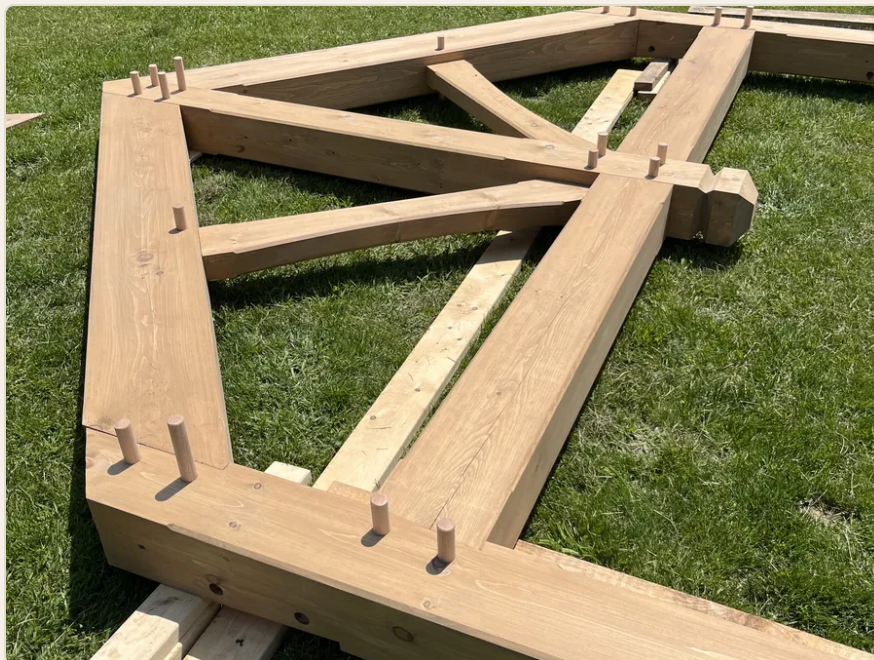
A SINGLE BENT, CUT AND DRY-FIT BEFORE RAISING — EVERY TIMBER SIZED FOR ONE JOB.
